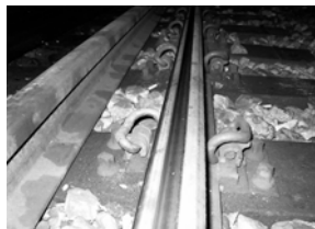
Fig. 4 – PANDROL fixing type using elastic clamps and PR3 un-deformed plate.
