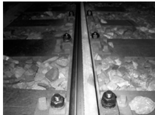
Fig. 3 – PANDROL fixing type using rigid grips and deformed PR3 plate.
