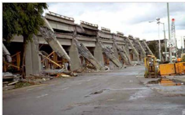
Fig. 2 – Cypress Viaduct - Loma Prieta earthquake, 1989.
